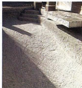
The steel is in for the perimeter bench, which allowed the cove to be eliminated. The floor was also raised.
