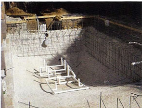
The shell prior to remodelling.
